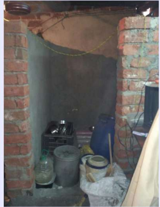
Ongoing toilet construction
